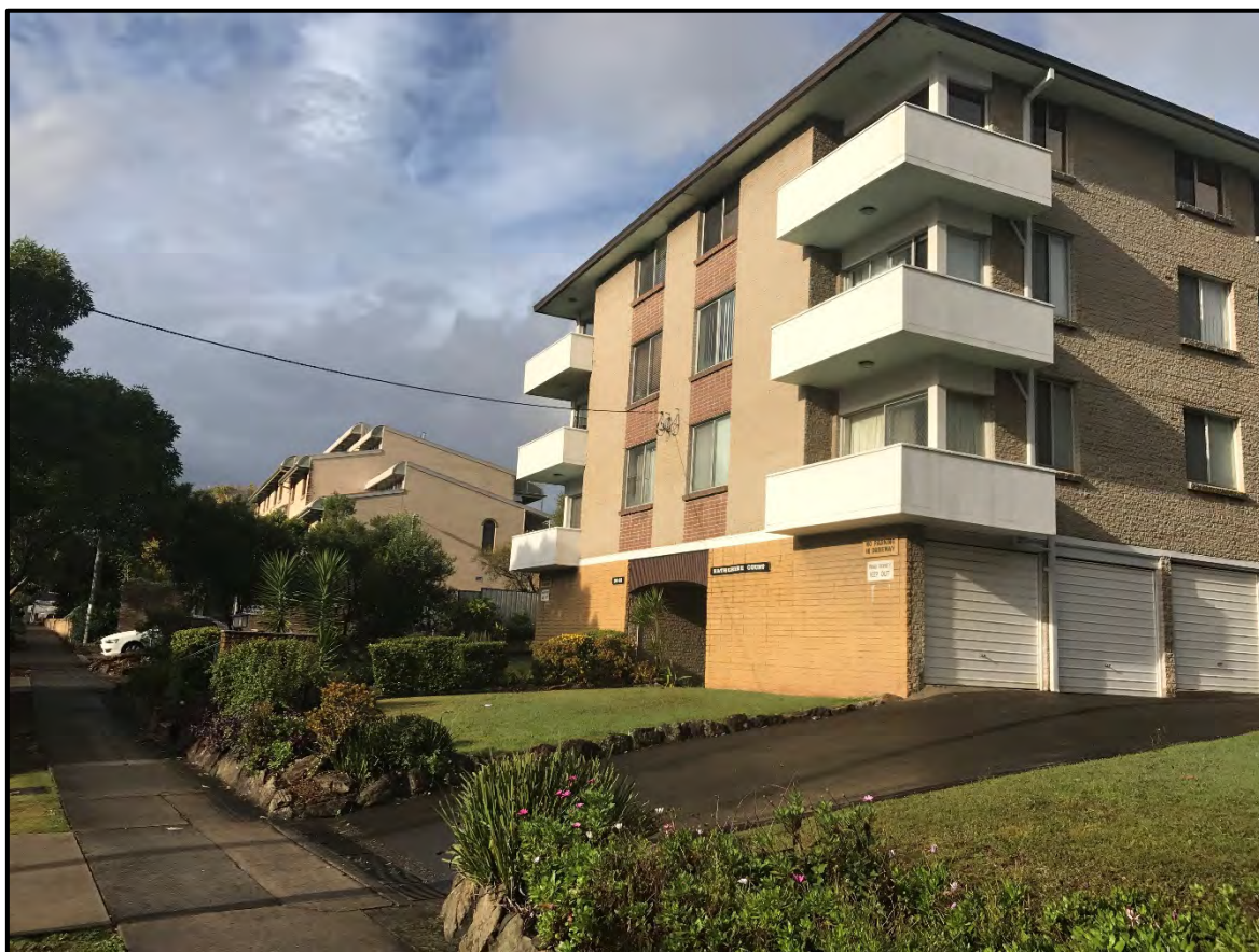
Figure 8: 4 storey residential flat buildings on the southern side of Padstow Parade
