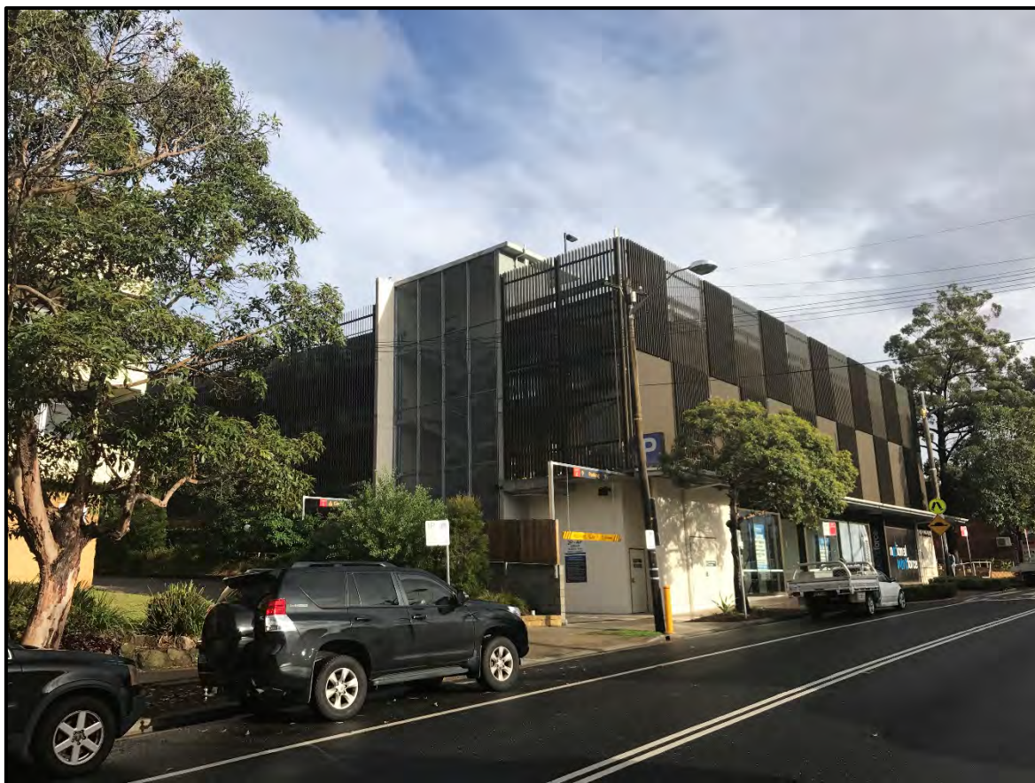
Figure 7: Recently completed four storey multi-storey car park on the southern side of Padstow Parade
